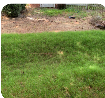
Structural Stormwater Conveyance
